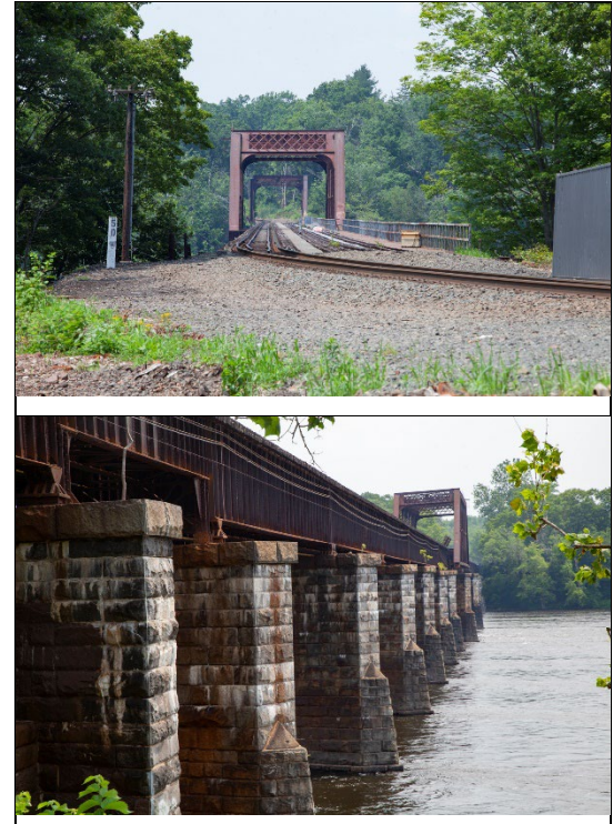
Connecticut River Bridge in Windsor Locks and East Windsor
