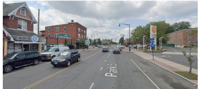
Approach to Parkville CTfastrak Station (Source: Google Maps)
