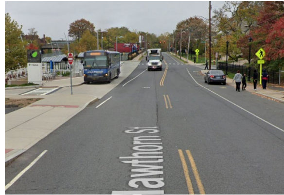
Approach to Sigourney Street CTfastrak Station
